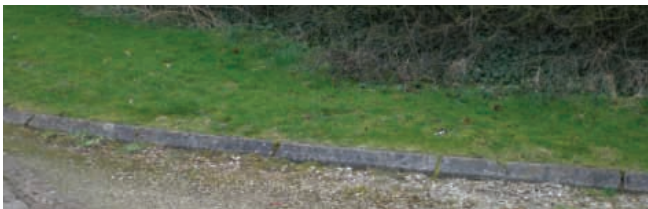
Concrete kerbs outside the electricity substation
