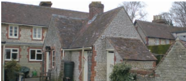
Outbuildings of number 4 Hethe Road Cottages
